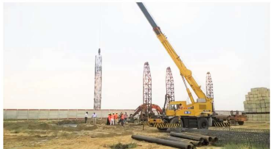
CONSTRUCTION OF PILES 241 NOS 900MM 4, 30M DEPTH COMPLETED IN 70 DAYS (2019) M/S. HINUCON (PVT) LTD, PILE FOUNDATION WORK AT PLOT #IT-03-A3 AND IT-04-A3 KORANGI CREEK INDUSTRIAL PARK, KARACHI.
