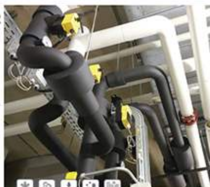
Flexible Closed Cell Elastomeric Thermal Insulation Foam
