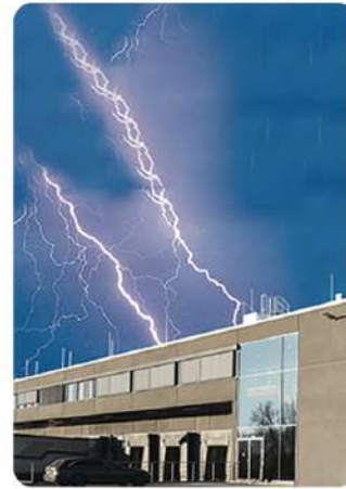
Lightning Protection System
