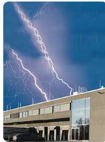
Lightning Protection System
